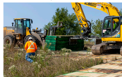
Below: A Stantec biologist inspects area to ensure there are no animals in harm's way before mats are installed.
