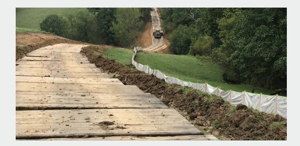
The Sterling site access team installed 14 miles of mats, safety protocols, BMPs, and culverted entrances to the county roads. They also implemented SWPP erosion control devices and cleared trees and brush to create access where none existed. On days of heavy snowfall, Sterling's work began at 4 a.m. with the opening up of county roads (blading off ice and snow), placing gravel, and cleaning off mats — all before the Michels team arrived at 7 a.m.
