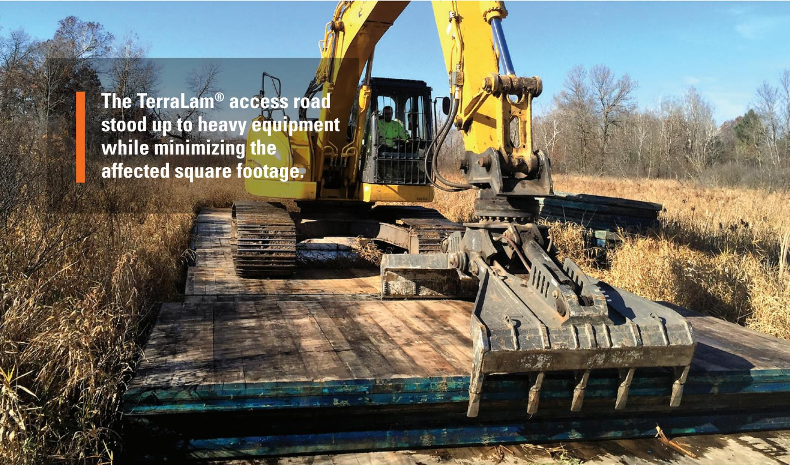
A yellow excavator is shown from a low angle, positioned on a narrow, temporary access road made of wooden planks (TerraLam). The excavator's arm and bucket are visible in the foreground. The background shows a field of tall, dry grass and trees under a clear blue sky.
